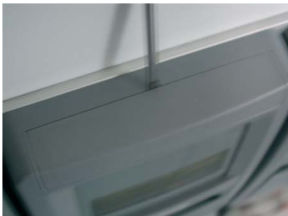
Removing tile to access the fastening screws
