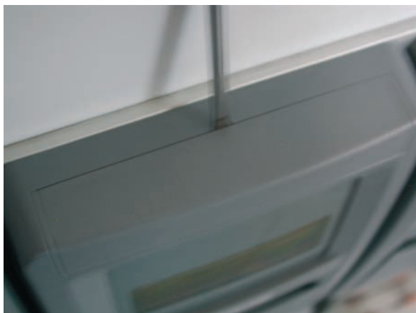
Removing tie to access the fastening screws
